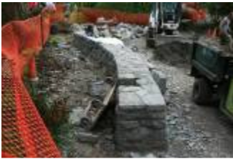
Photos by R. Girton showing path and wall construction at CSRG.
